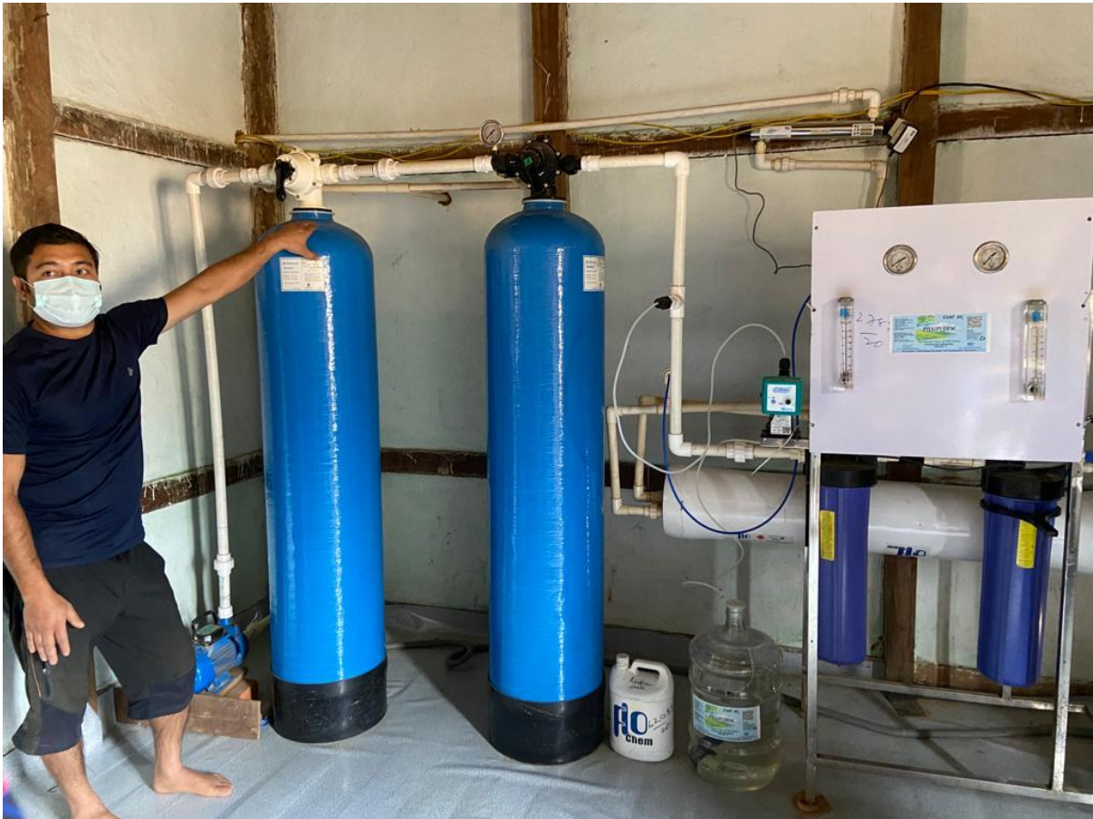
Touring the Local Community drinking water at Chandonpokpi(Phaipei ),Phaipa Dew
